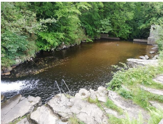
Figure 2-4. Sediment built up between Cathole Falls and a manmade weir
