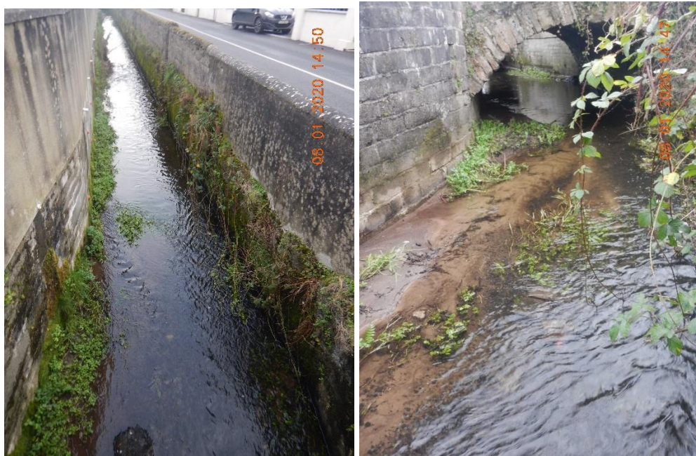
Figure 2-13. Showing extent of channelisation and vegetation growth observed at toe of bank (left) and fine sediment deposition observed on inside bends, toe of banks, and around structures (right)
