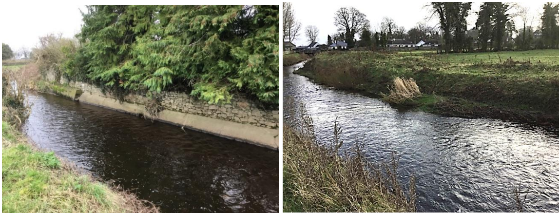
Figure 2-9. Signs of bank degradation in Owenass 3 include ad-hoc concrete and possibly historic town defences (left), and signs of historic poaching and slumping (right)
