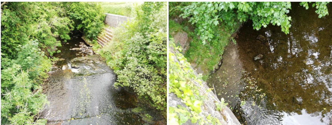
Figure 2-5. The bed of the channel in Owenass 5 exhibiting signs of instability through incision of bridge aprons (left) and siltation of the bed substrate (right)
