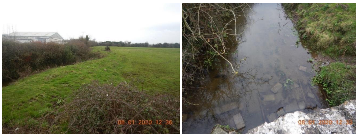
Figure 2-15. Low embankment beside river shows signs of previous dredging/maintenance works (left), with fine sediment deposits observed on bed (right)
